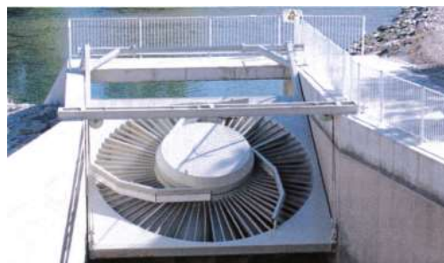
Photo 15 : Turbine VLH (source : MJ2 Technologies)
